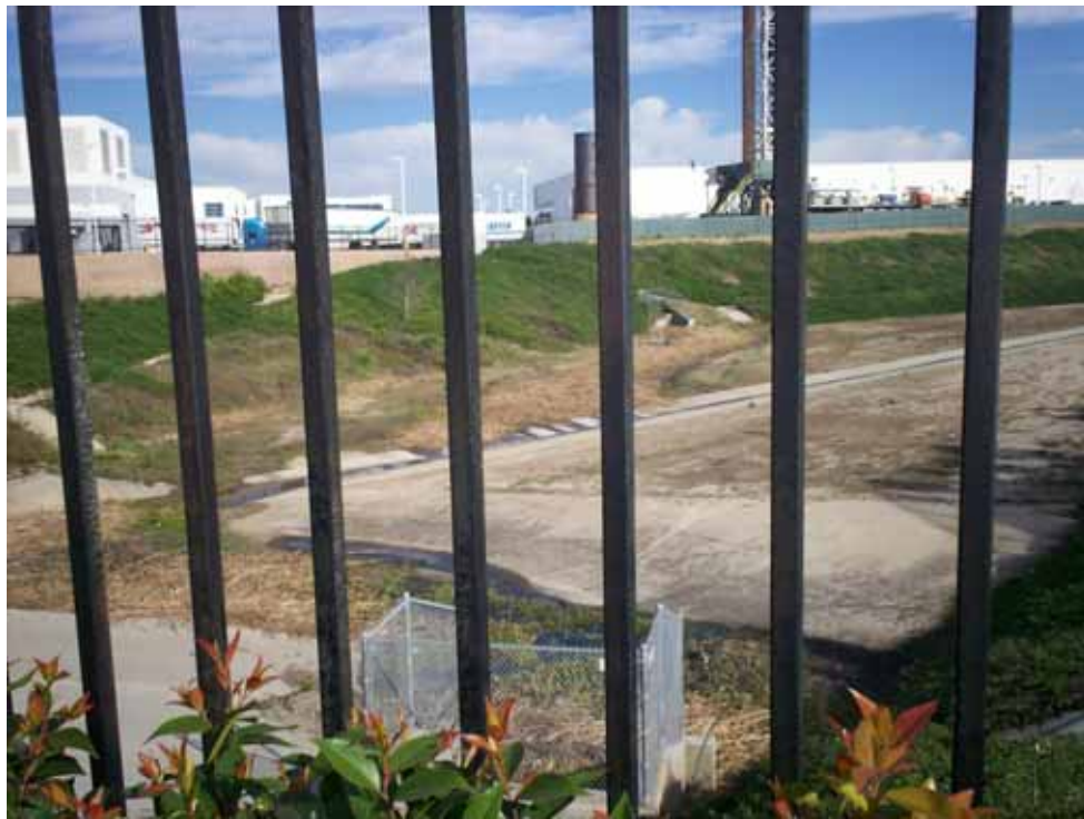
Photo 7: Outfall with ponding and cattails in stormwater basin sediment deposit, facing north-northeast from fence along Beachey Place
