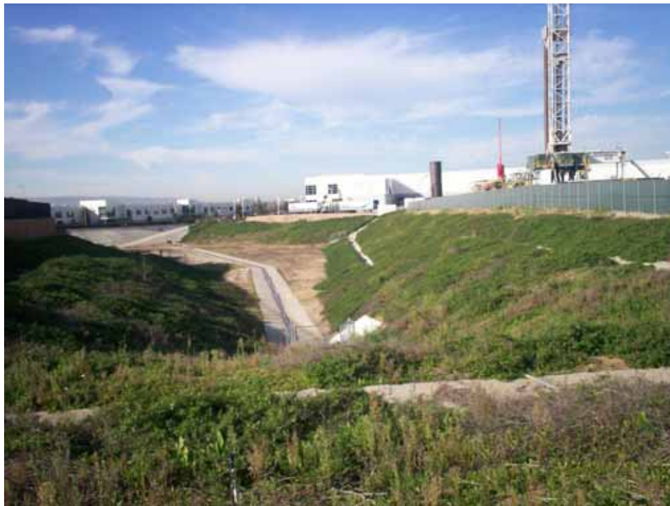
Photo 5: Stormwater Basin, facing west-southwest from fence along Bishop Avenue. Oxy site photo right.
