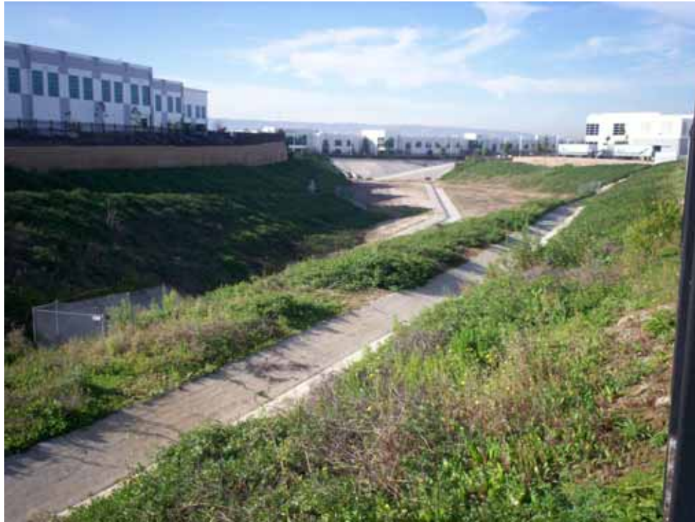
Photo 3: Stormwater basin, facing southwest at fence along driveway of 18030 Bishop Avenue (approximate address)
