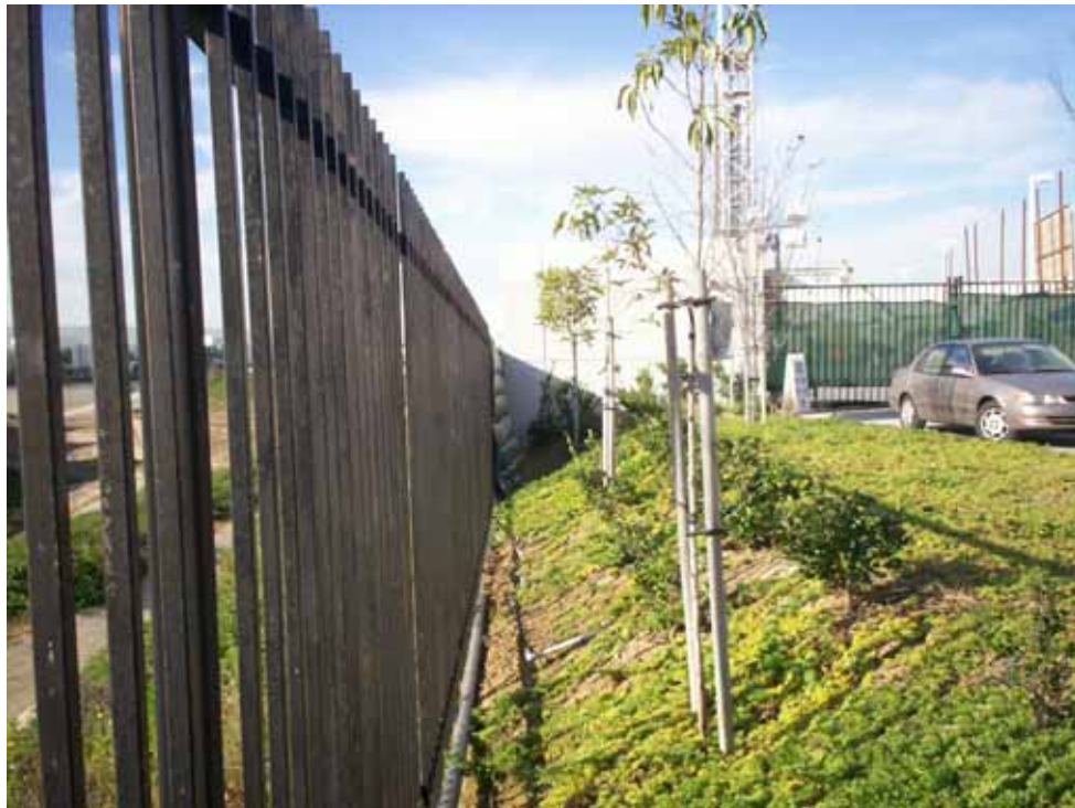
Photo 4: Fence at stormwater basin along driveway of 18030 Bishop Avenue (approximate address), facing west. This is one driveway entrance to the Oxy site.
